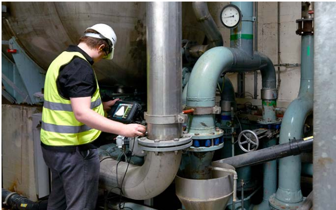
Industrial pipeline inspection with Proceq Flaw Detector 100
